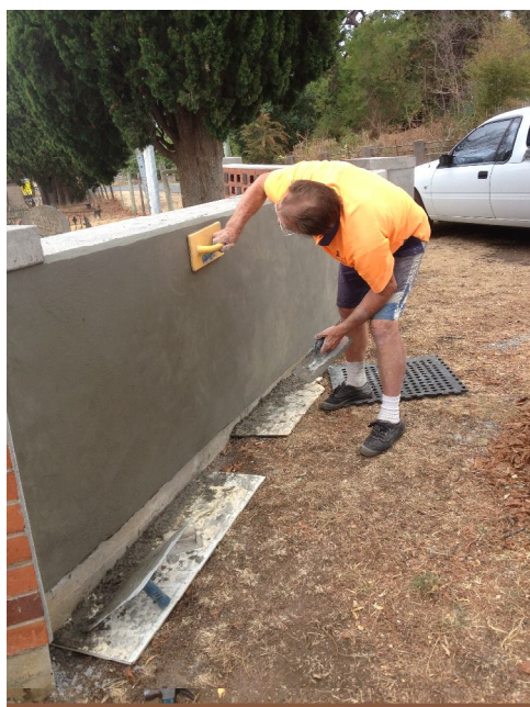
Joe Mennen works on the rendering of the Columbarium Wall at St Matthias' Church in Windermere Road.
